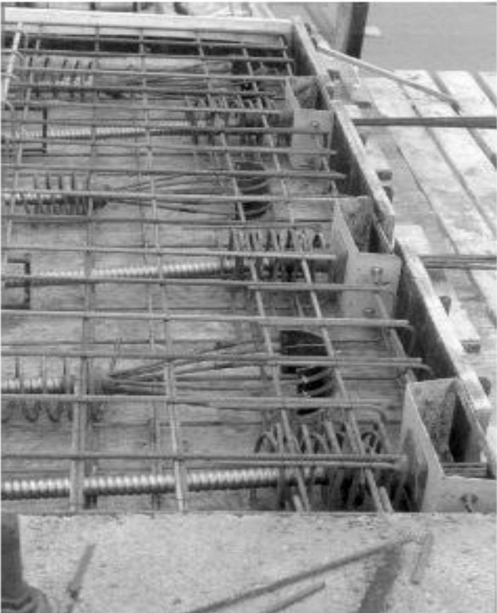
Figure 1.1: Anchorage provide for the safe introduction of post-tensioning forces into the concrete.
