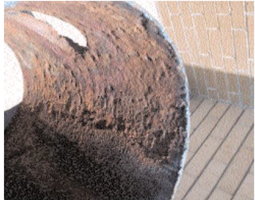
Hydrochloric Acid and Hydrogen Sulfide Corrosion
