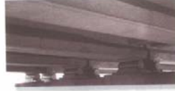
Rollers and associated bearing pads are used to support the prestressed concrete girders of a highway bridge.
