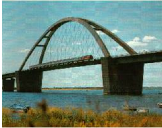
Figure 14. Tied Arch Bridge.
