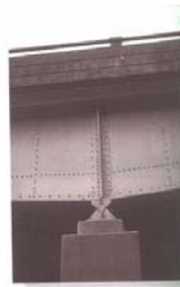
Typical pin used to support the no girder of a railroad bridge.
