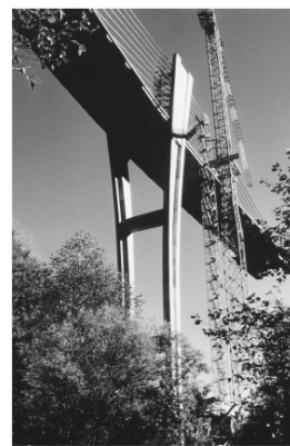
FIGURE 3.6 Christian Meiss's Sannberg Bridge.
