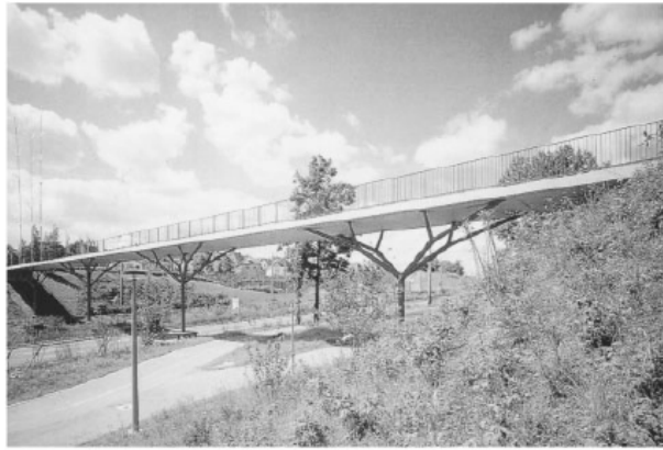
FIGURE 3.4 One of Jorg Schlaich's footbridges.
